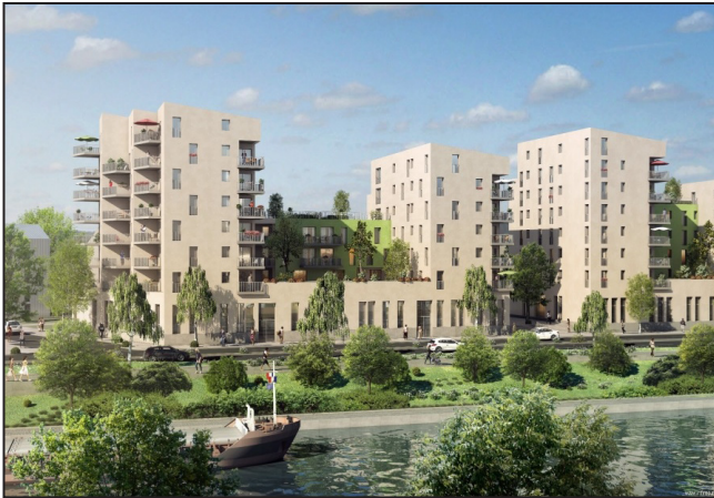
Fig 74: Investment property offered to landlords by Akerys in the Paris region of 2 room 37 sq m flats for €169,000 6
