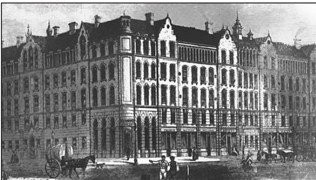
Fig 19: Peabody Trust's first estate in Commercial Rd 1863 1
